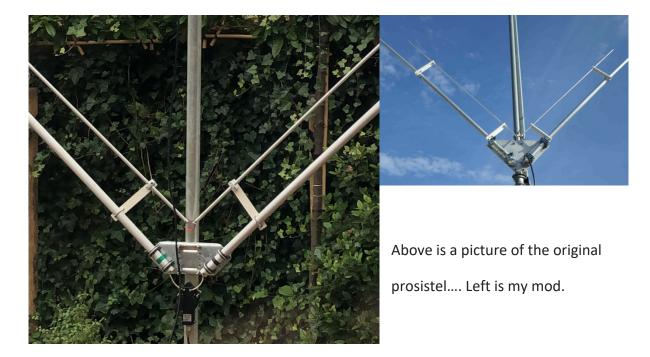
Connect the centers together with a piece of 1.5 or thicker alu / copper wire, or a strip of copper.
